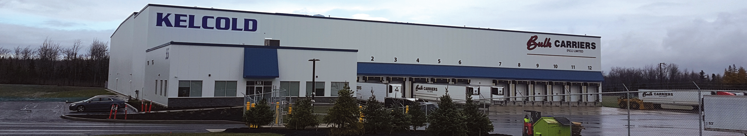
Kelcold's 101,000 square foot, third-party cold storage facility in Caledonia Industrial Estates handles all types of frozen food, from dairy products to meats. PHOTO: CONTRIBUTED
